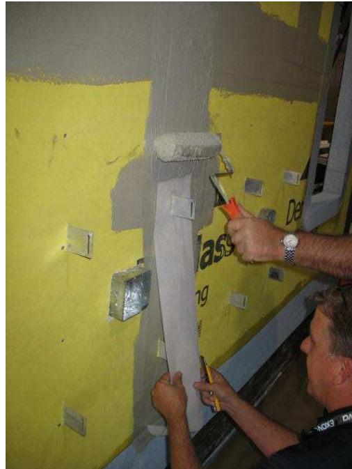
Figure E-5 – Application of LATICRETE Waterproof/Anti-Fracture Fabric along Sheathing Joint / Brick Ties
