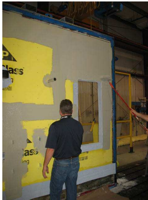
Figure E-6 – Application of LATICRETE Air & Water Barrier
