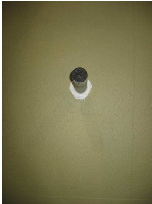
Figure E-12 – Application of MVIS Silicone Sealant around PVC Pipe
