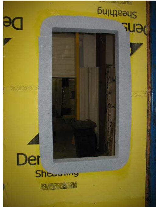
Figure E-1 – Application of LATICRETE Flexible Sealing Tape around Window Rough Opening
