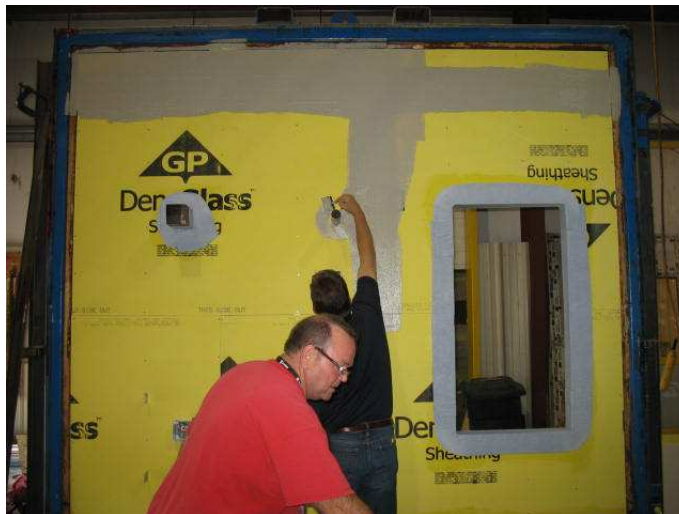
Figure E-4 – Application of LATICRETE Air and Water Barrier
