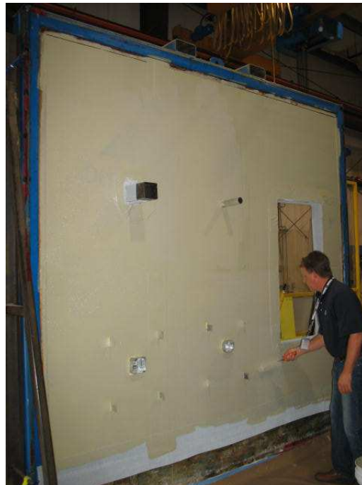
Figure E-8 – Application of LATICRETE Air & Water Barrier
