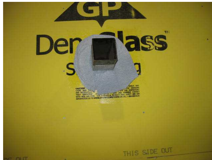
Figure E-2 – Application of LATICRETE Flexible Sealing Tape around Duct
