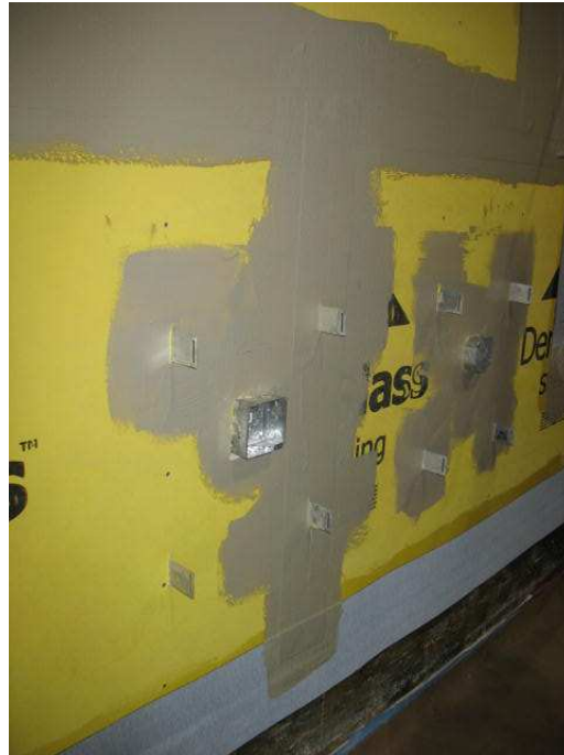
Figure E-7 – Application of LATICRETE Air & Water Barrier
