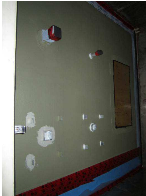
Figure E-13 – Completed Wall Assembly (red Tuck Tape along Foundation Interface used for Extraneous Bagging Purposes)
