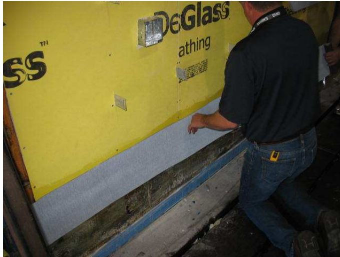
Figure E-3 – Application of LATICRETE Flexible Sealing Tape along Concrete Foundation Interface
