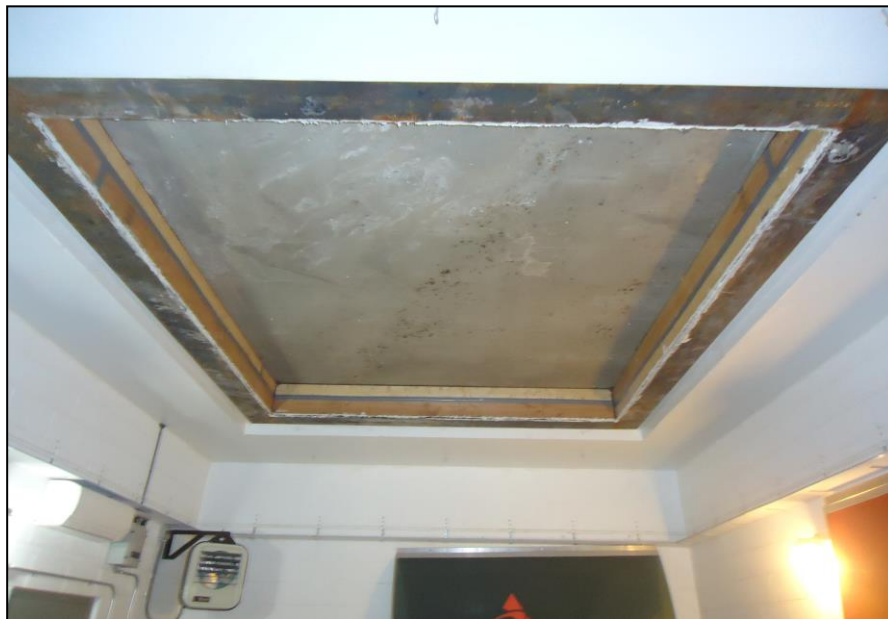
Source Room View of Test Specimen Installation
